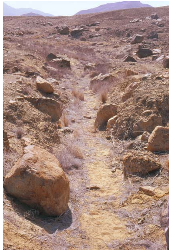
Water Management in Peru. Fig. 8 Ground view of the hydraulic control structure upstream of the chute and Hoya Hondada aqueduct. Photo by C. R. Ortloff.
